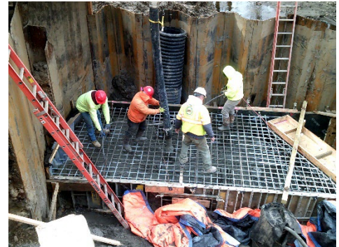
Essex County, Dougal Bridge Replacement
