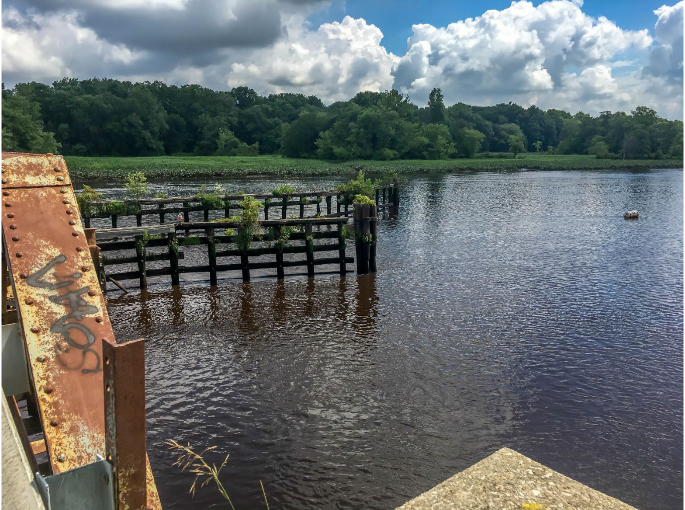
Centerton Road Bridge Demolition, Burlington County
